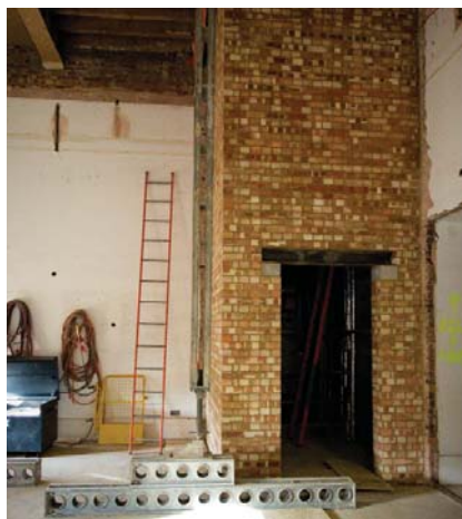
The new lift shaft viewed from the first floor
