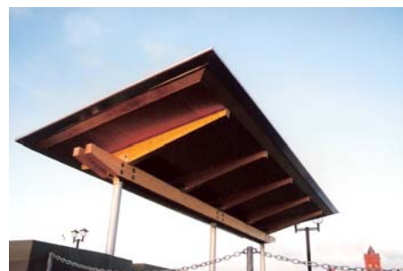
Figure 4: Cantilevered Timber Beams
