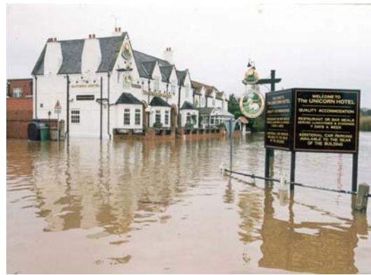
Figure 2: Impact of localised flooding
