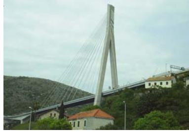
Figure 2: Cable Stayed Bridge
