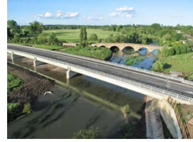
Figure 3: Reinforced Concrete Bridge with masonry arch bridge in background
