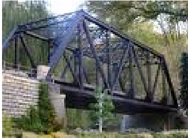
Figure 4: Steel Truss Road Bridge
