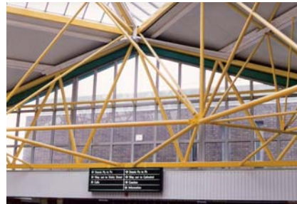
Figure 5: Space Frame Roof Structure
