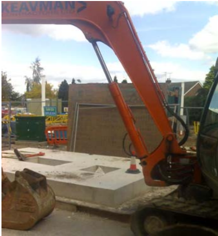
Fig 1: Typical slab cast ready for lifting
