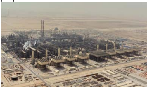
Figure 2: Pearl GTL – largest construction site in the industry
